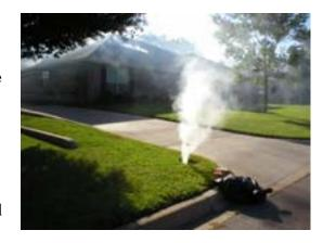
Pipe, connections and seals of the wastewater drain system in and under your building are damaged, defective, have clean out plugs missing or are improperly installed.
