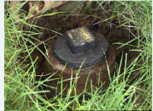
Typical sewer cleanout with properly installed plug.
